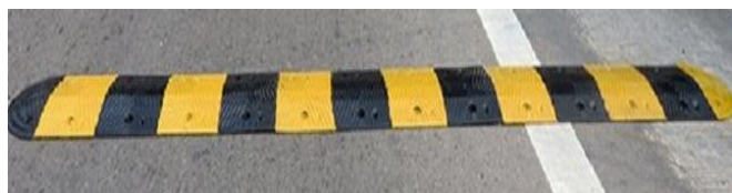
Fig. 7. Sine-shaped speed bump
